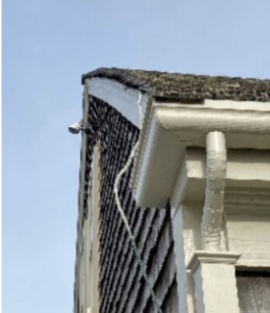
Slightly Bowed Roof
