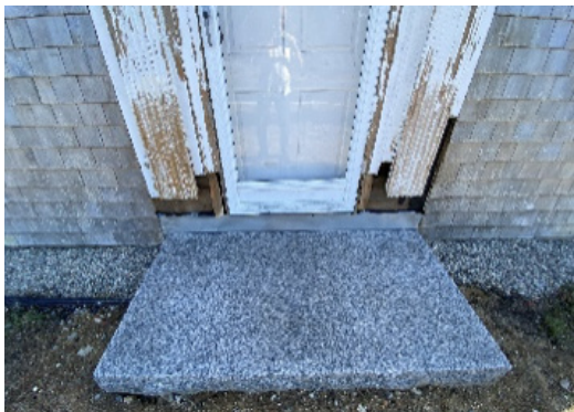
Decayed Pilasters
